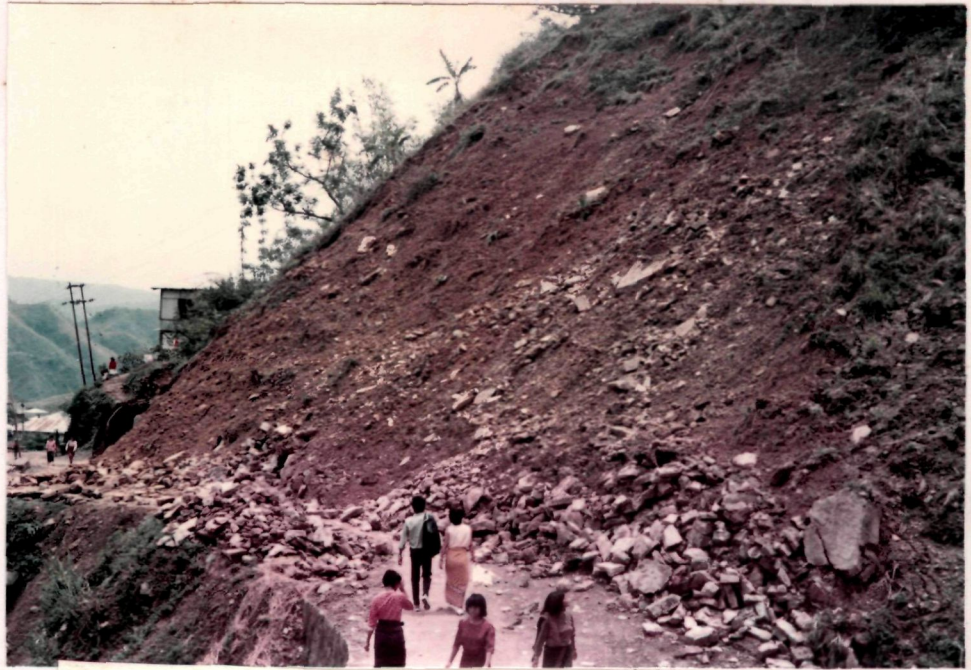
PLATE NO. 8 : Major landslide on a loose sedimentary formation at Bethlehem Veng.
