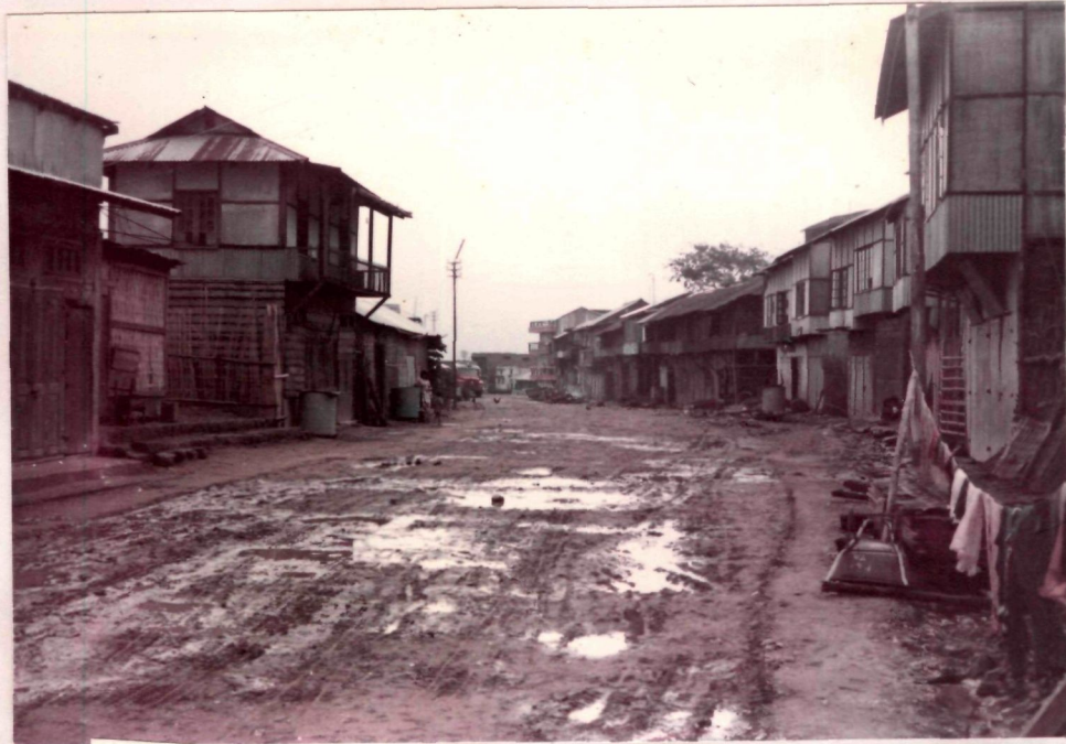
PLATE NO. 28: Champhai street; a typical house type in growing towns of Mizoram.
