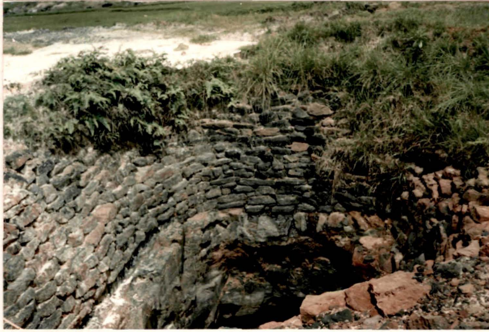
Plate 1.1a - Pit formed as a result of 'rat hole' method of mining on the plain surface
