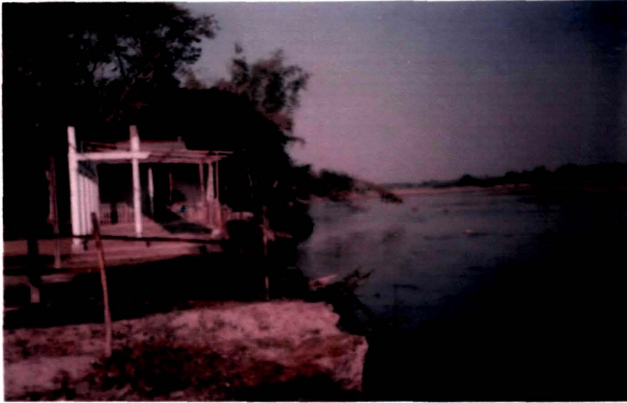
Plate 7 : A Kali Mandir is seen in devastating condition due to bank erosion
