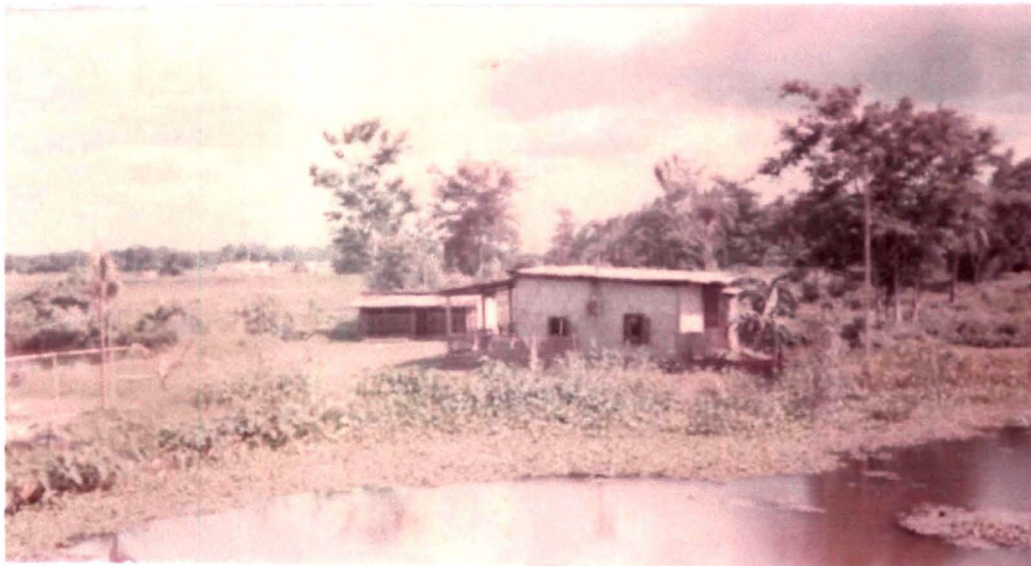
Plate 6 : A Mosque under temporary shed which was displaced due to flood, 1984
