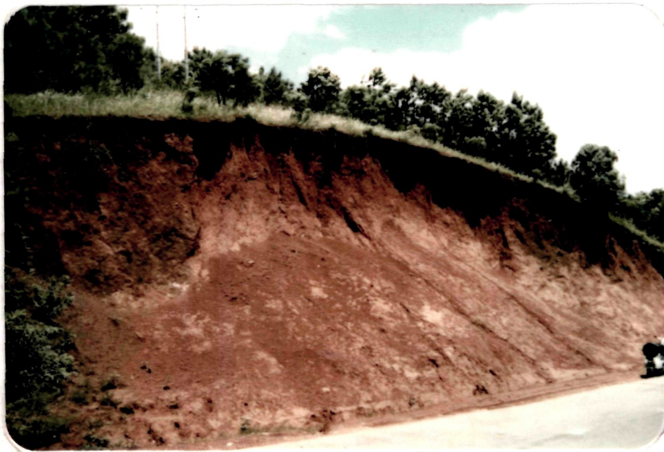
(Plate-7) : Landslide (slump) along slope profile (steep cuts) in soil after Khasi Greenstone.
