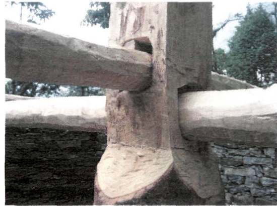
Carved poles for traditional house under construction
