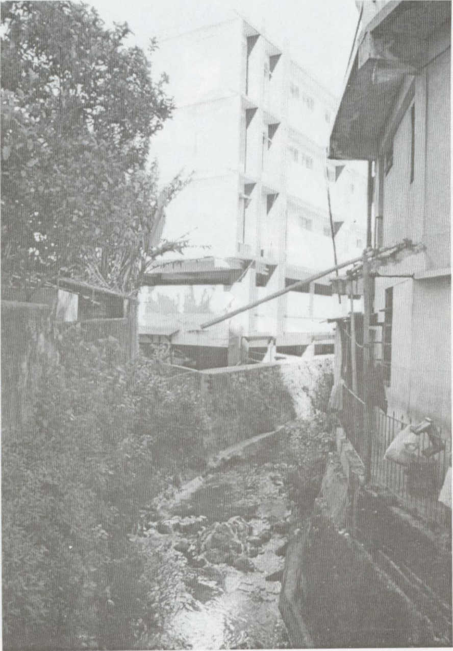
Contaminated liquid waste released from Bethany Hospital into the adjacent stream.
