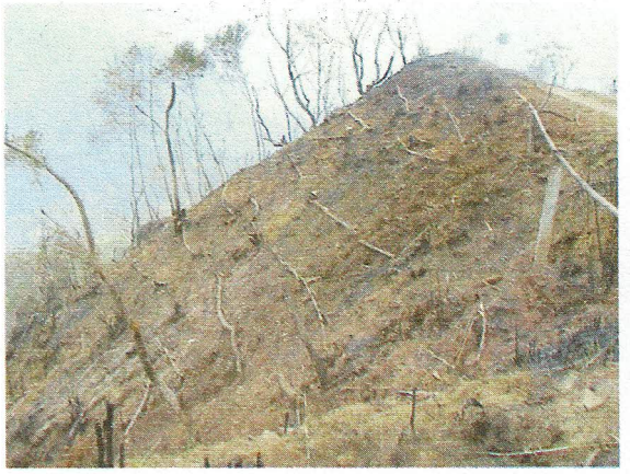
Plate 1.8 : Poles laid across the slopes in staggered manner.
