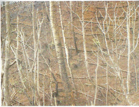
Plate 1.8 : Poles laid across the slopes in staggered manner.
