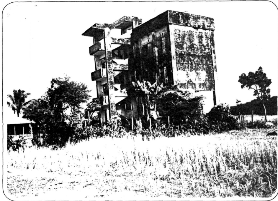
Cyclone shelter near sea beach
