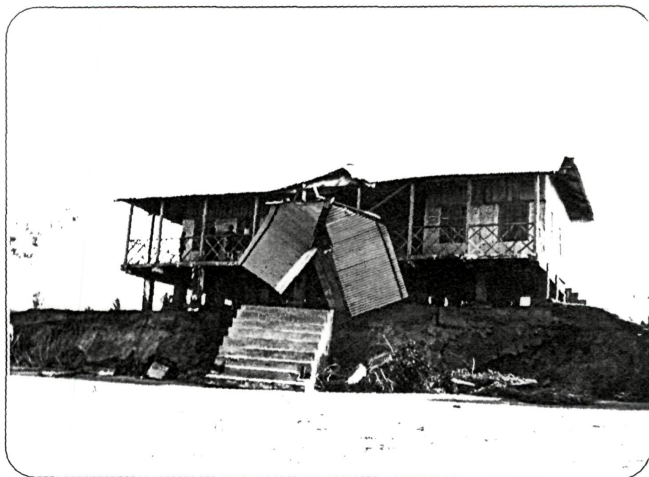
Government guest house damaged by sea wave
