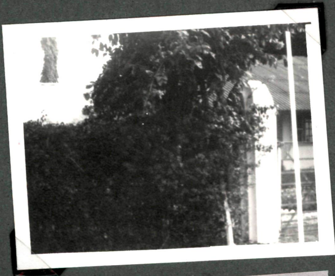
A side view of Dakmoka Inspection Bungalow.
