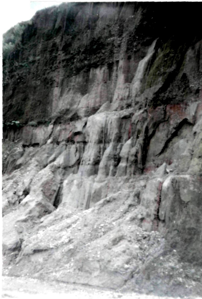
Jointed rock mass Landslide prone zones along road cuts
