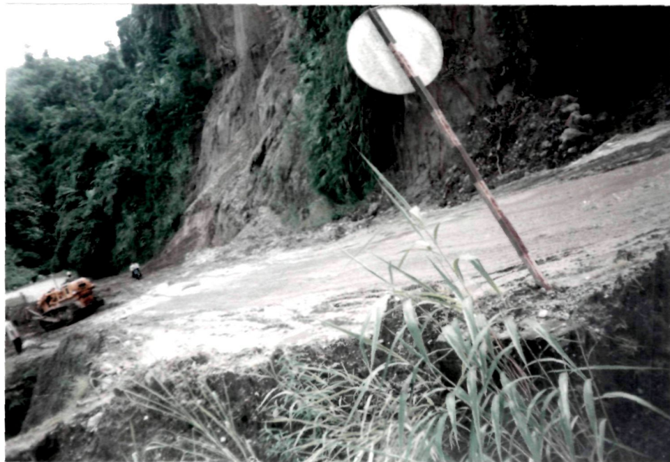
Jointed rock mass Landslide prone zones along road cuts
