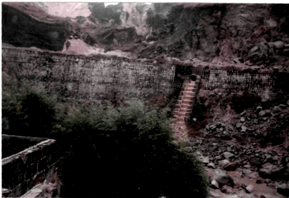
Fig. 4.07 : View Showing the Sediment Outflow From the Quarry Site into River Umtyngar. The Quarry Site is at the Right Bank of the River.
