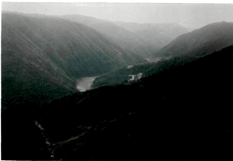
Fig. 4.01 : View of Umiew River Up-Stream of On-Going Works of Dam Across the River
