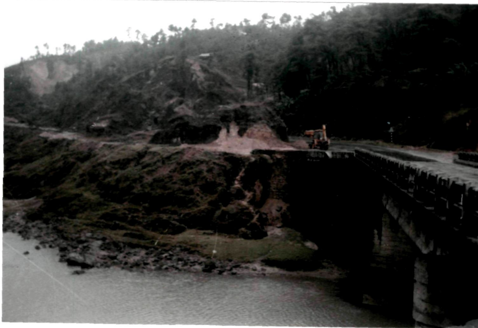
Fig. 4.06 : View Showing Sand Quarry Operation by the Excavator at the Right Bank of River Umtyngar Along Shillong- Sohra Highway
