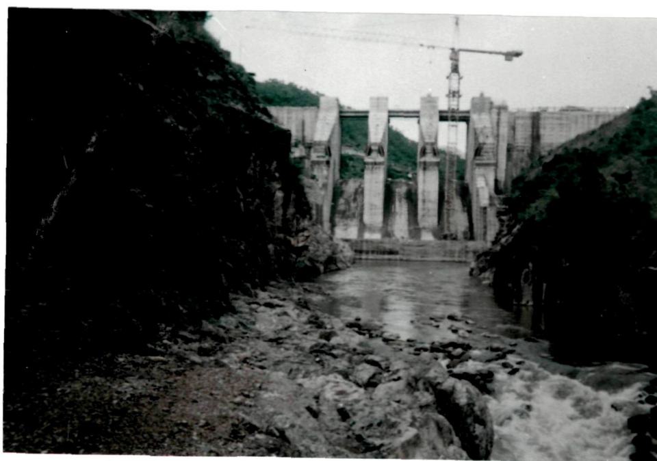
Fig. 4.02 : View of Umiew River Down-Stream of On-Going Works of Dam Across the River
