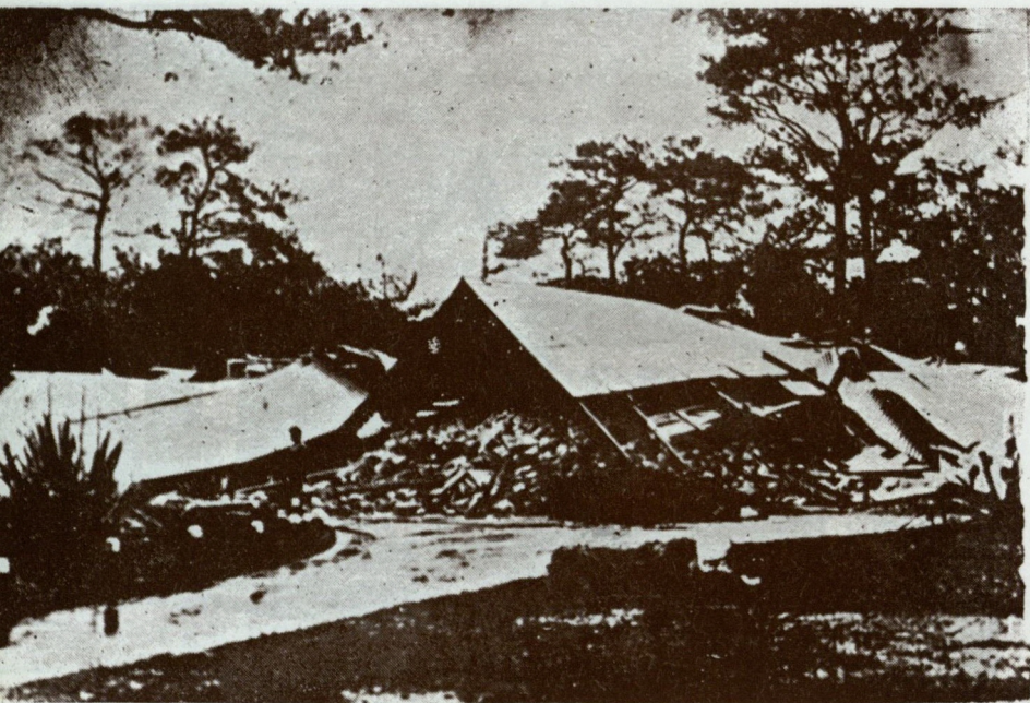
The ruins of the Chief Commissioner's residence after the earthquake of 1897.
