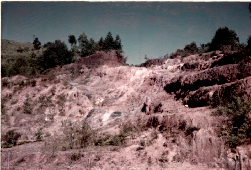
Plate No. 4 Hillslope being bulldozed near Janapih
