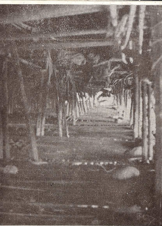
Interior of Lokku (destroyed by earthquake) Moshup
