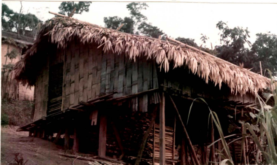
PLATE NO.4.8 : A typical Riang house is made up, except for the poles, completely of bamboos.
