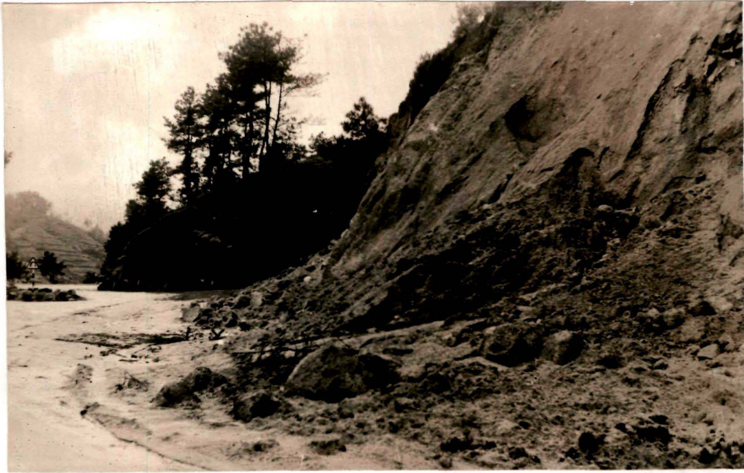
Debris fall along Shillong-Cherra road. (Photo taken 5 minutes after the fall)
