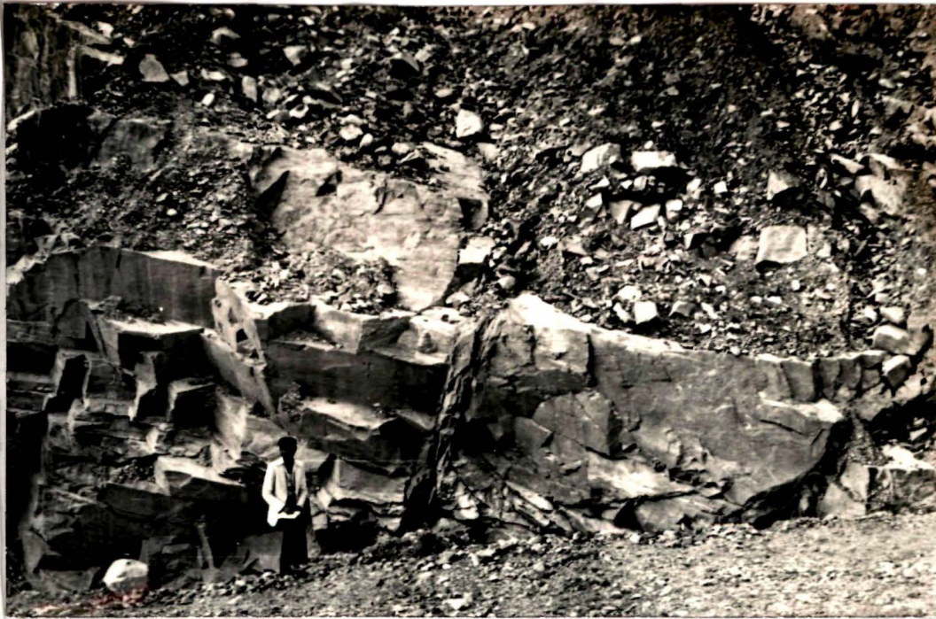
Rock sliding. Note the shape & size of the rock pieces
