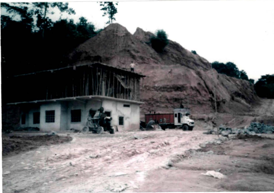
Plate 20b Cutting of slopes for constructional purposes (human settlement).
