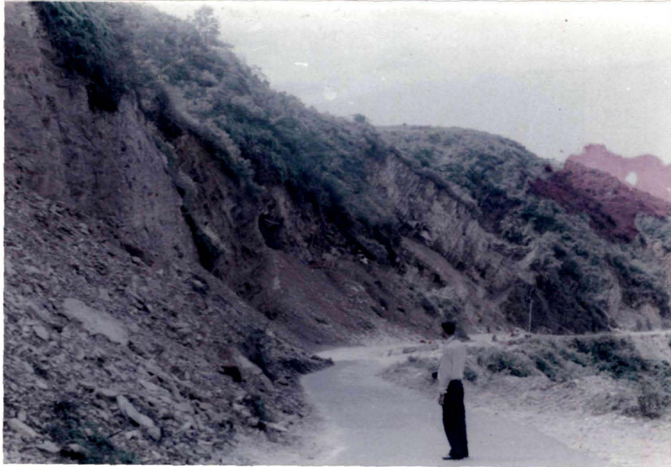
Plate 19 Abrupt steep slope cuts of more than 60^\circ all along road networks have made the slope profile unstable.
