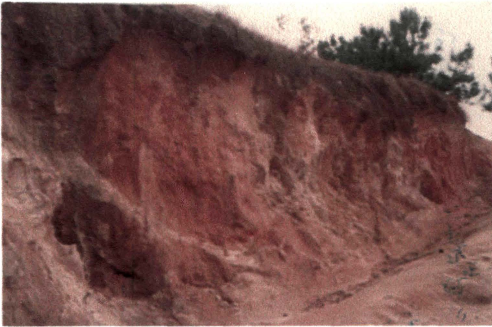
Plate No. 3 - ROADSIDE CUTTING AT KYNRUD
