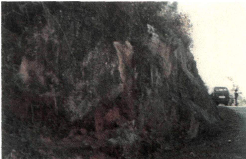
Plate No.6 - ROADSIDE CUTTING AT KYNRUD EXPOSING QUARTZITE
