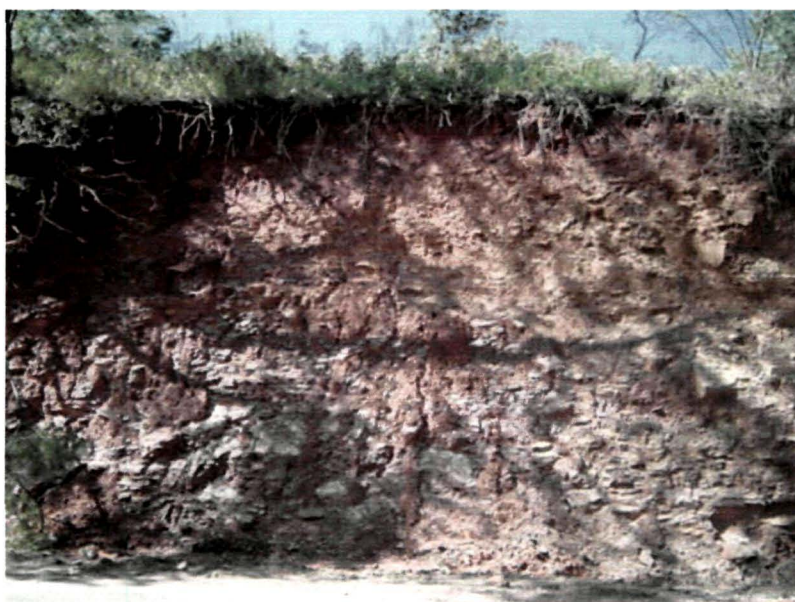
Figure 3.47: Partial weathered soil of B horizon overlying bed rock (Quartzites).
