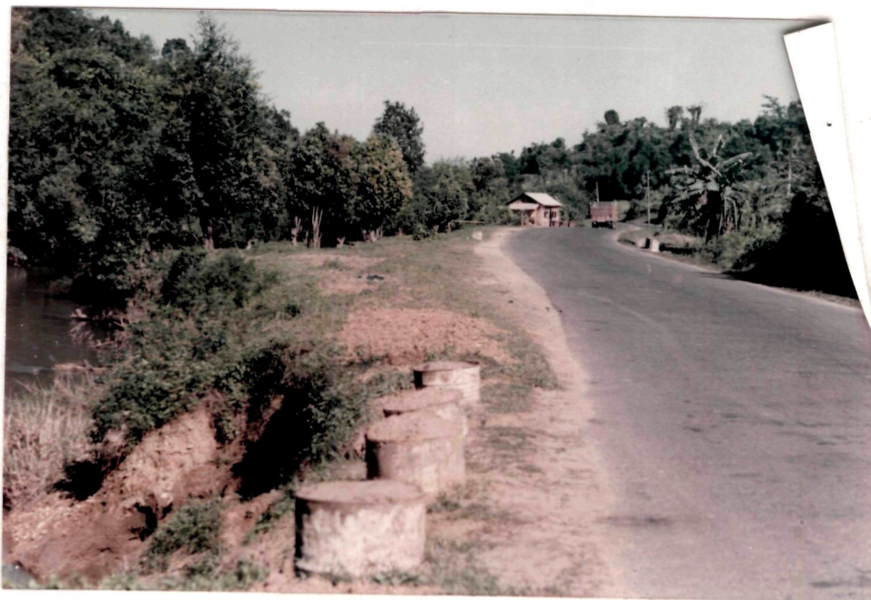
Plate 6(a): Roadside settlements cause a lot of disturbance to traffic movement and these are mostly food stalls, which attract a lot of customers, specially truck drivers. This results to parking on the roadside causing great inconvenience to movement of traffic.
