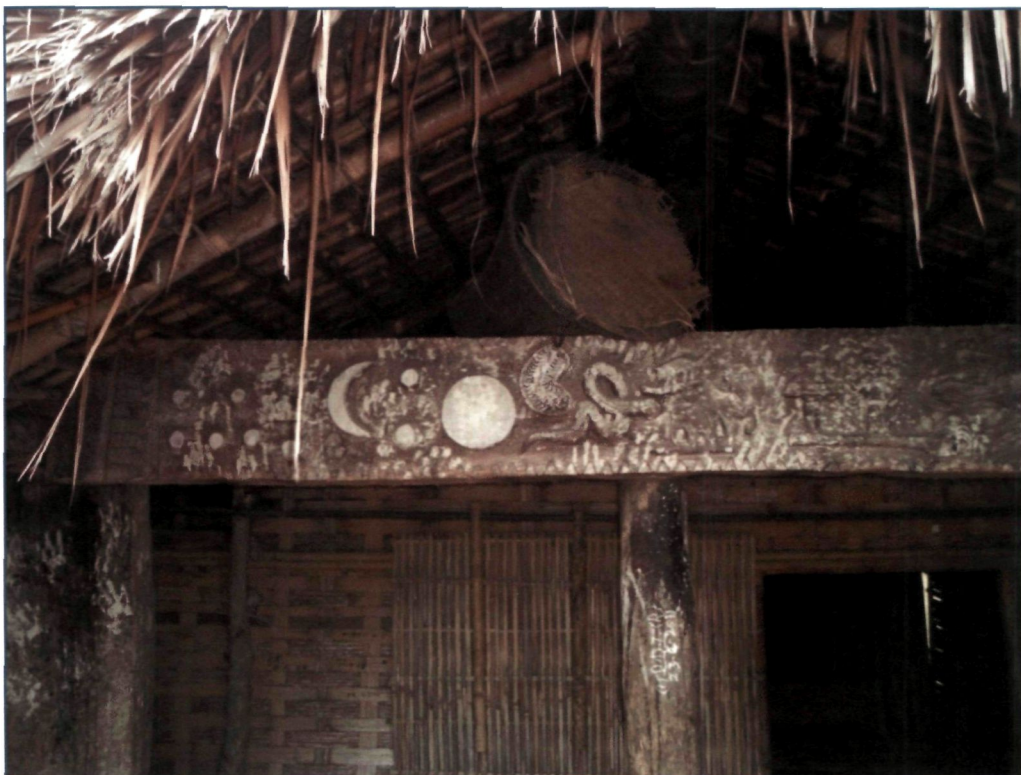
Fig. 55 The front carved beam of a nokachik called a bilbang . (other crossbeams are also called bilbang )
