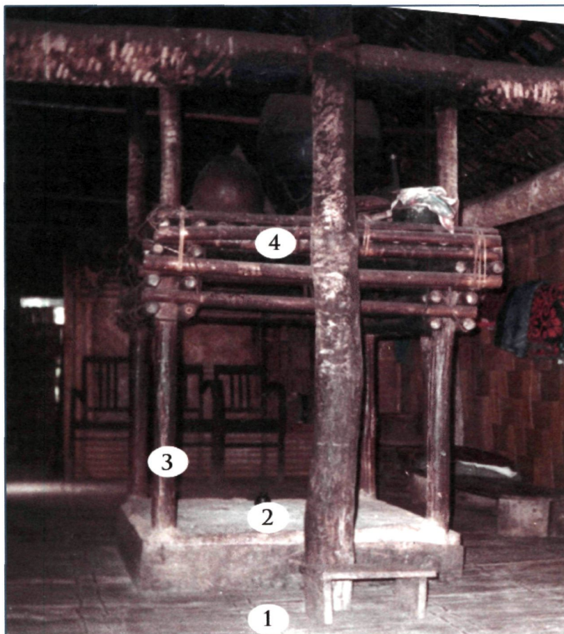
Fig. 115 Parts of the onggal/bilbang area 1. Chuchekra 2. Hearth 3. Dangknok 4. Ongari 2.
