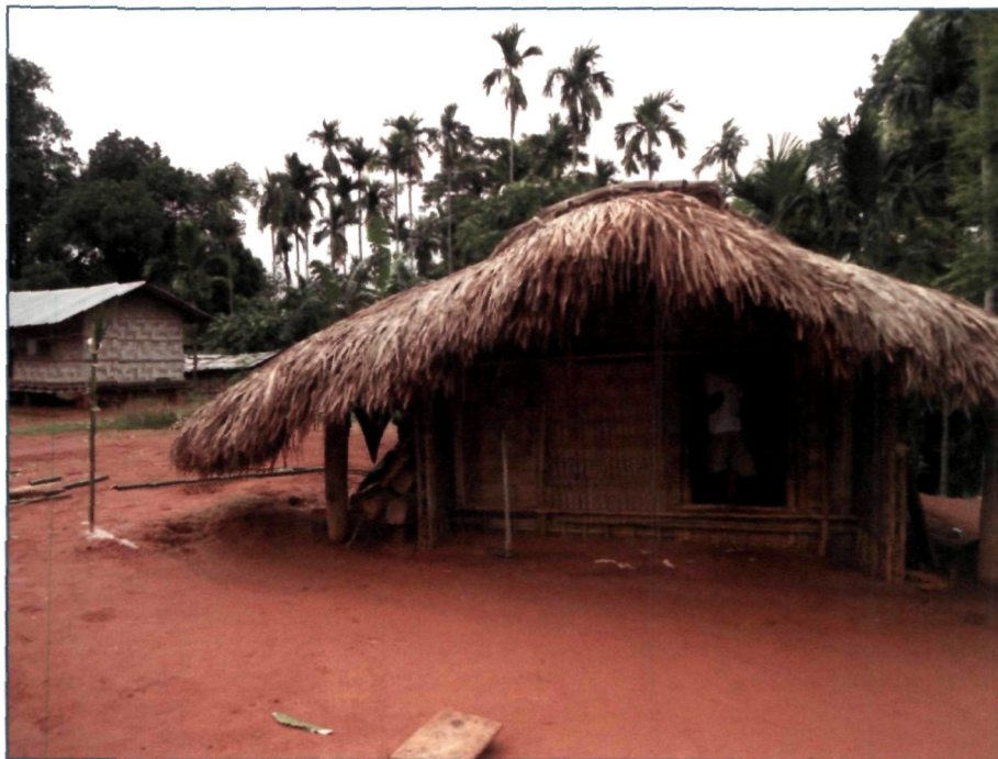
Fig. 49 Front view of a nokachik . The part under the roof is called the ballim and the roof covering it is called the pangsoni . The bamboo with the egg is erected to the right if the child is male and to the left if the child is female.
