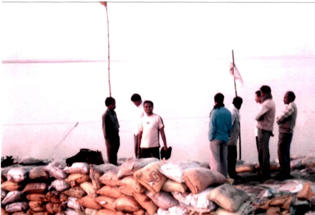
MEMBERS OF EROSION PROTECTION SANGRAM SAMITTEE WITH SAND FILLIG BAGS
