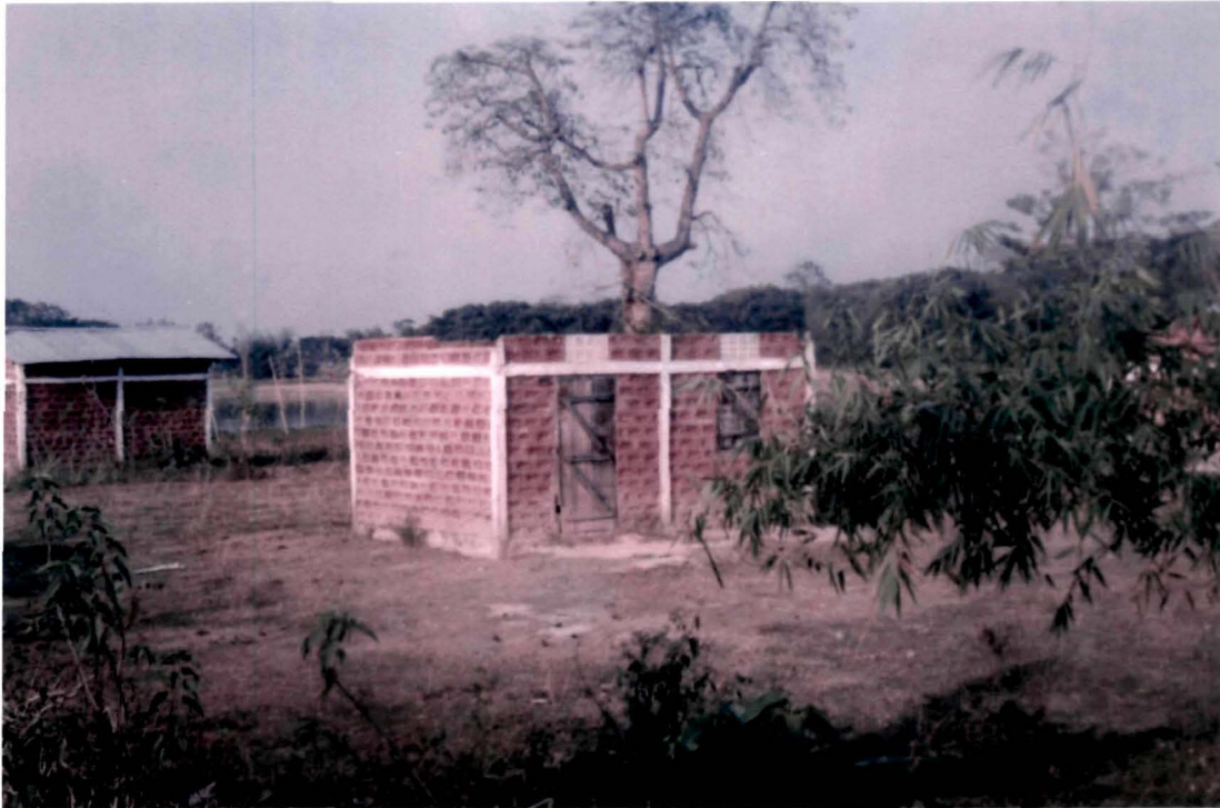
HOUSES PROVIDED TO AFFECTED FAMILIES UNDER INDIRA AWAS JOJANA
