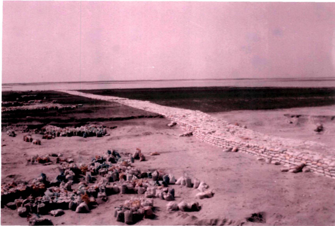
SAND SPUR CONSTRUCTED BY LOCAL PEOPLE IN BHURAGAON
