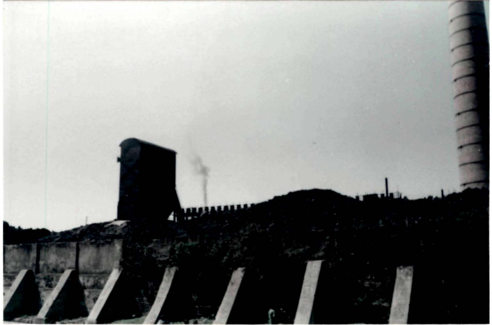
Plate - 12 Stack gases coming out of Coke Plant
