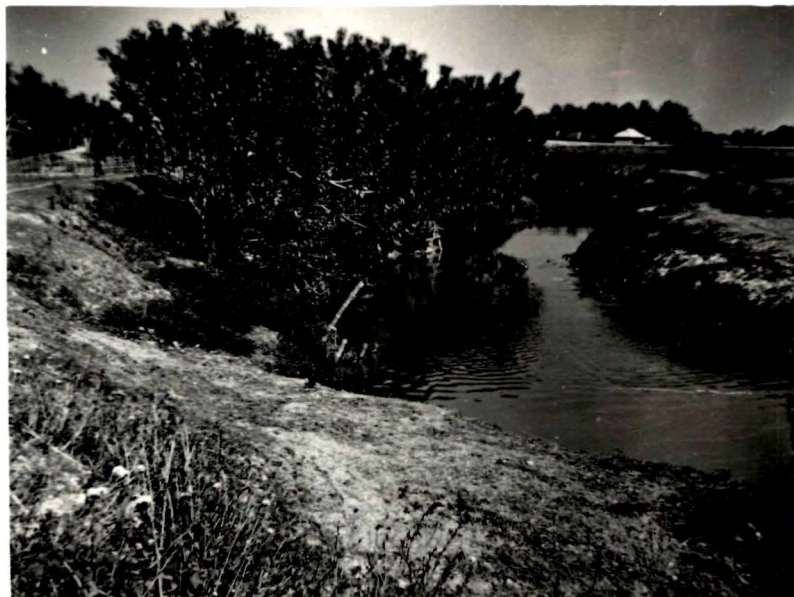
4. The nature of gully erosion by a tributary of Haora river.
