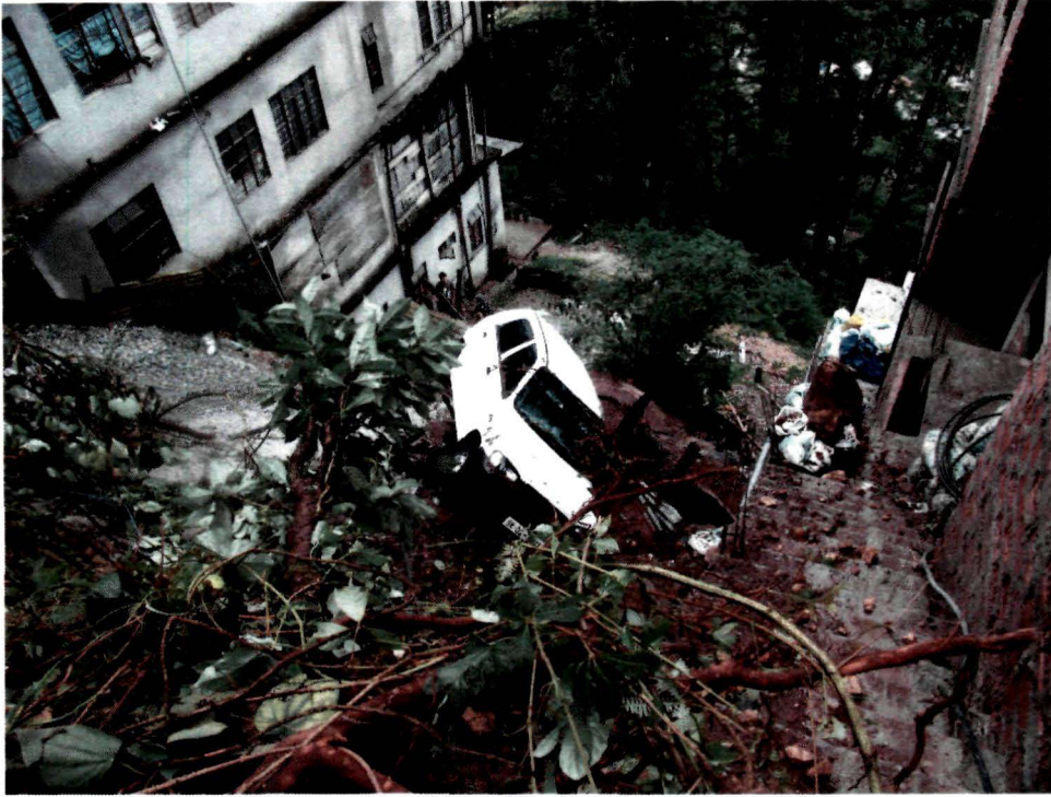
Plate 11 House and property damaged by minor landslide
