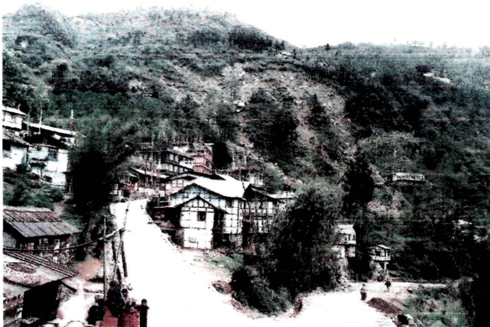
Plate 9 A major landslide near Chandmari in 1997 (Courtesy: Bhasin, et al.)
