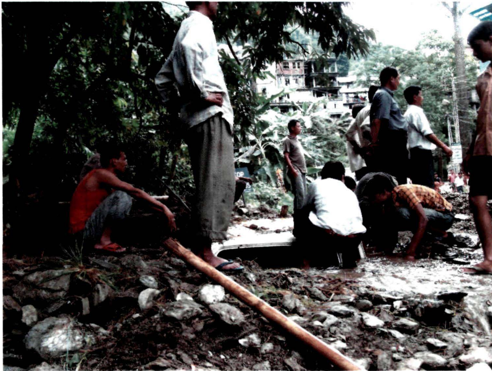
Plate 12 Vehicle under the debris of landslide
