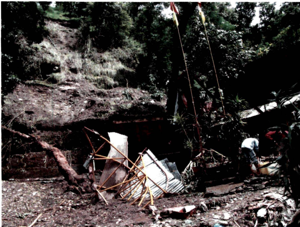
Plate 16 Landslide near 6 th Mile locality
