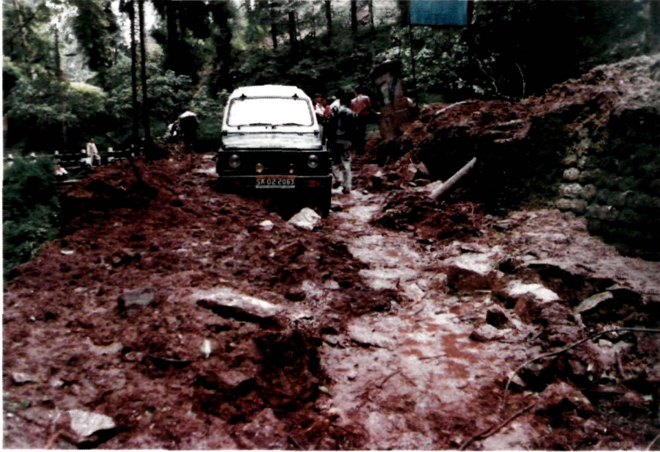
Plate 15 Road blockage due to landslide
