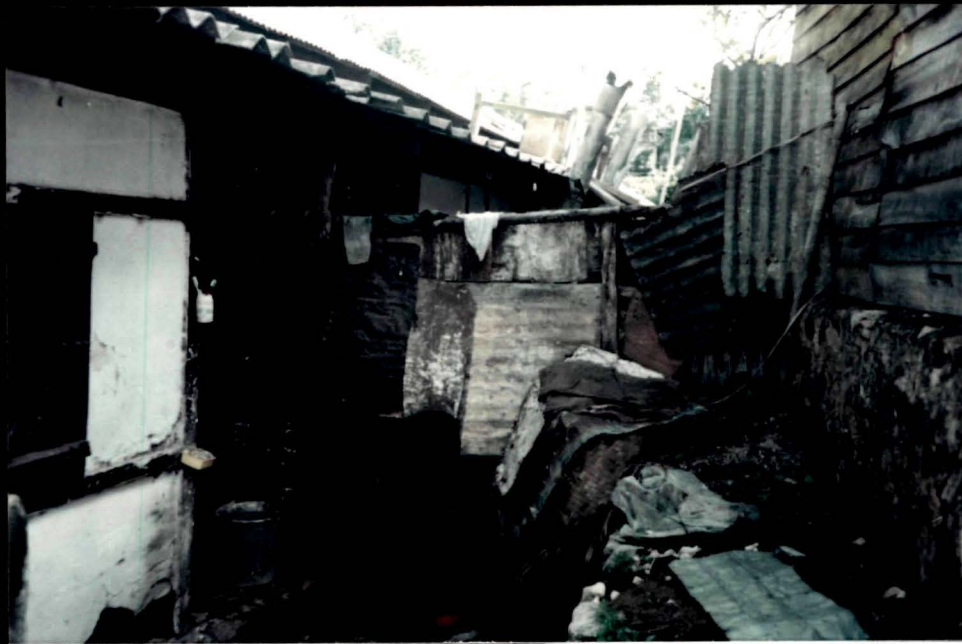
4.3 Typical dwelling of the urban poor (Sweeper Colony, Laitumkhrach)
