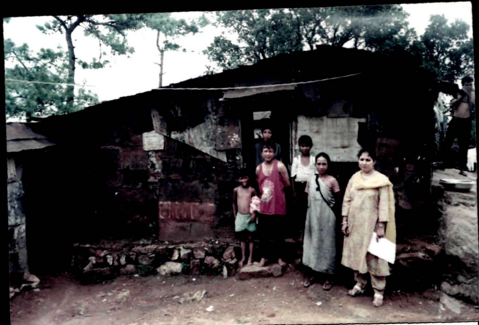
4.7 Dilapidated housing condition of Khasi slum dwellers (Upper Lumpharing)
