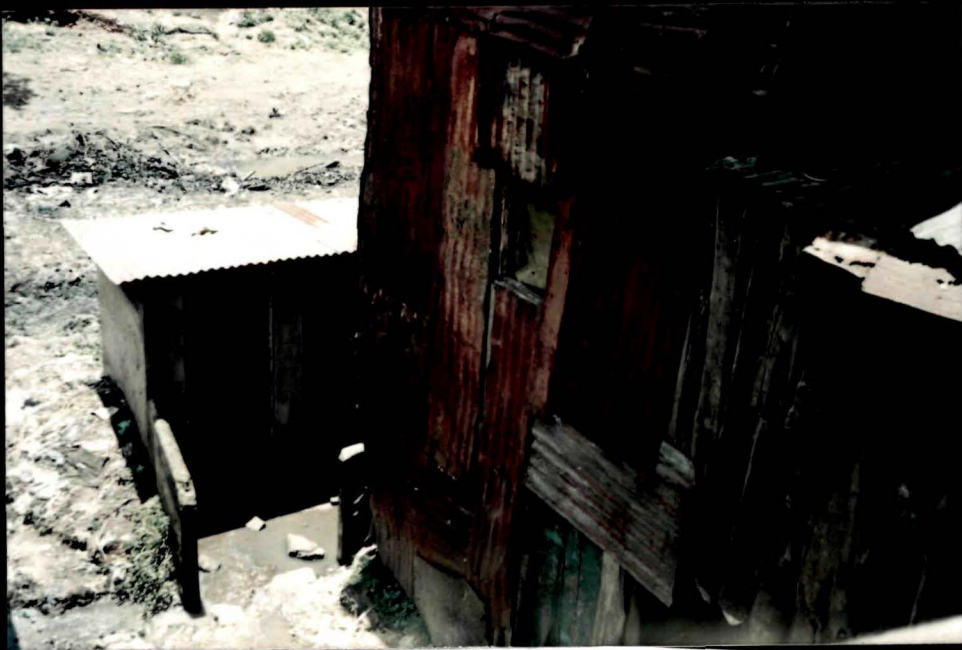
Building Materials are scrap tin sheets
