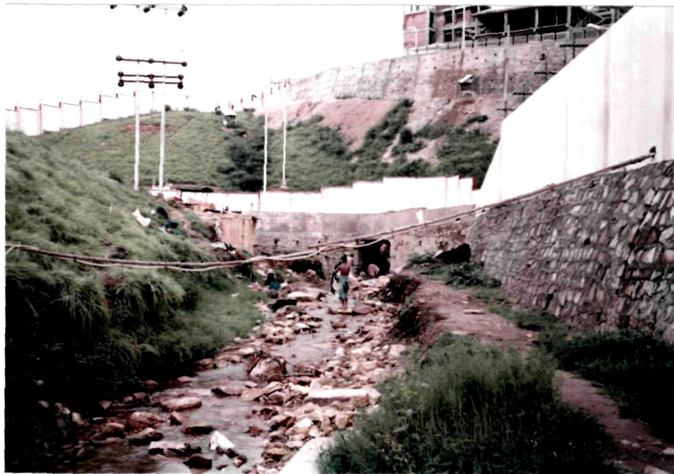
6.11 Construction of Office Complex at Lapalang Water Source
