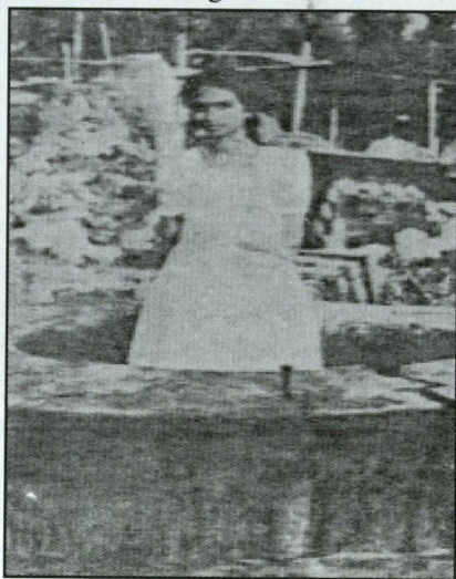
Photo 1 Choked well in Jorhat town in Purana Masjid (Poddar, 1952)
