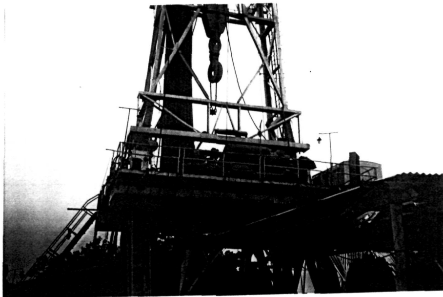
20. A view of a drilling rig of ONGC, ERBC.
