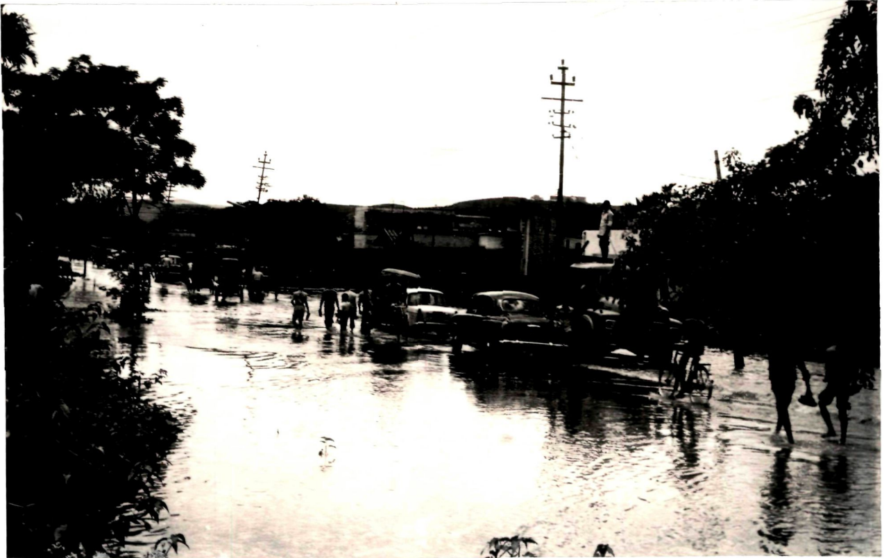
Plate 10: Overflows of rainwater on R.G. Baruah Road.
