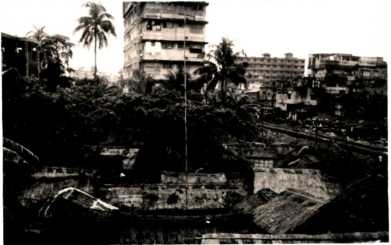
Plate 16: A slum pocket near Panbazar Over Bridge, Guwahati.
