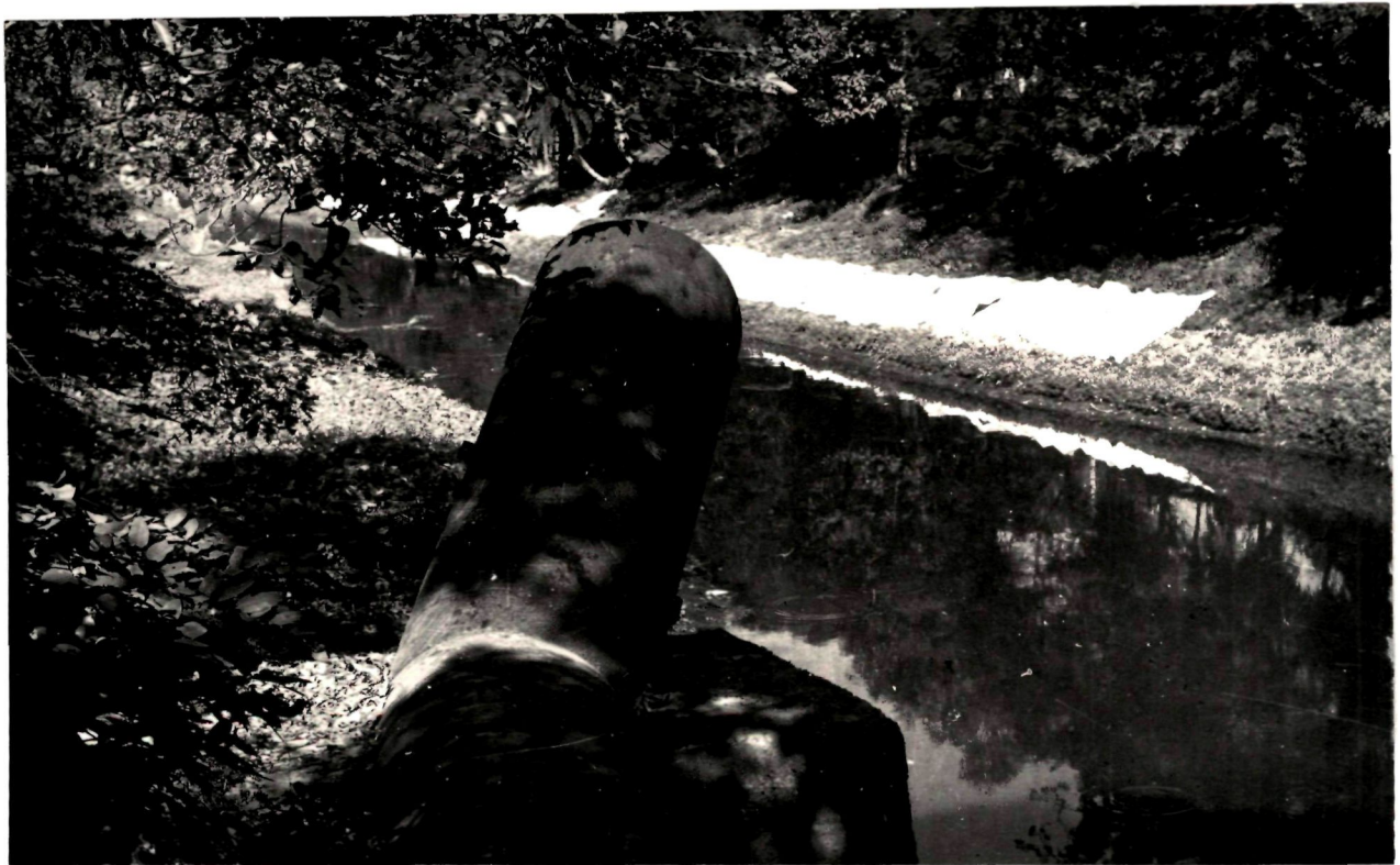
b) The pipe line by which excess inundated water pump out after closed down the sluice gate of Bharalu river in front of Pragjyotish College.
