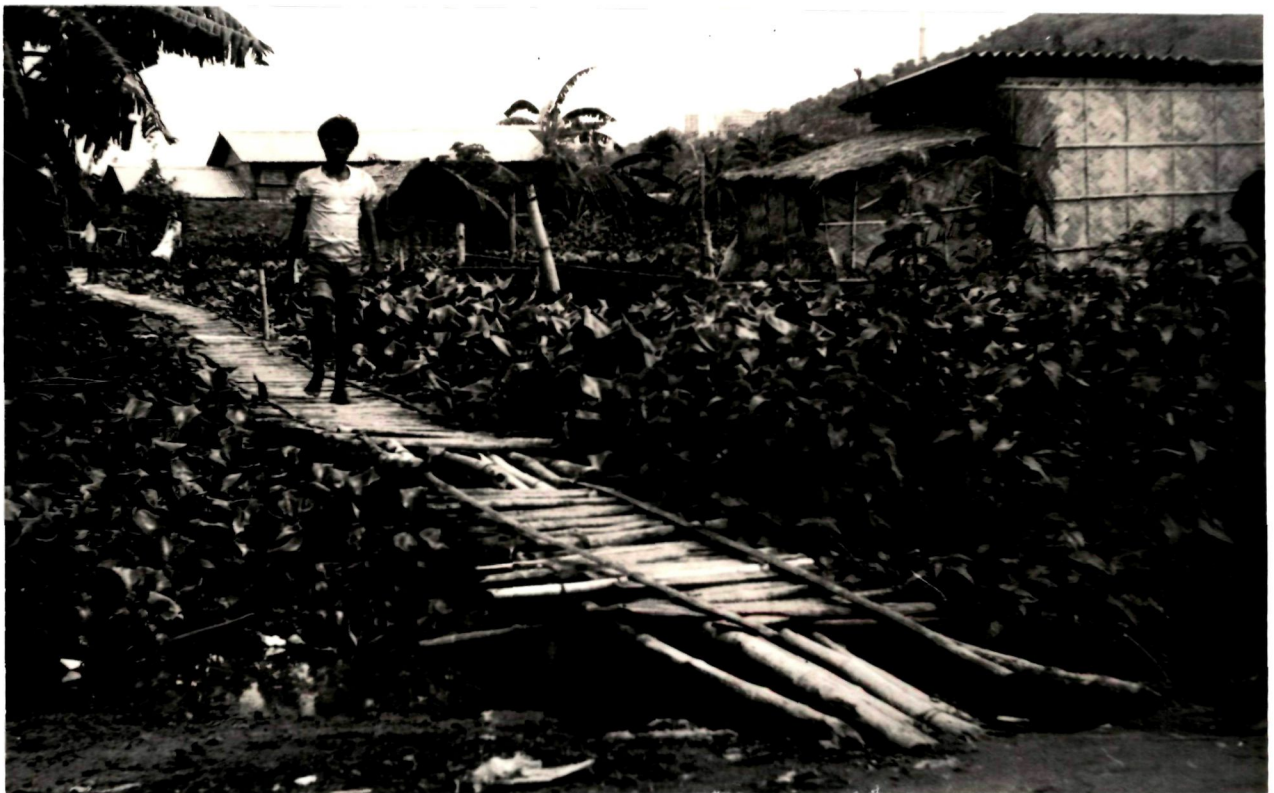
b) Same area of (a), here they constructed bridge of bamboo to approach their houses.
