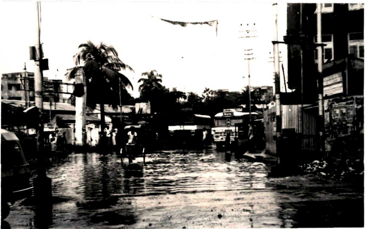
Plate 8: Waterlogged road between the State Police Reserve gate and Ram Mandir.
