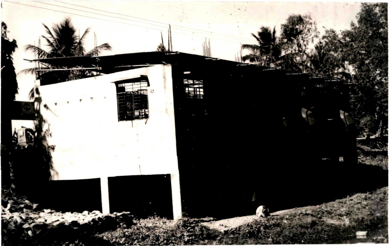
a) Pumpset power house
