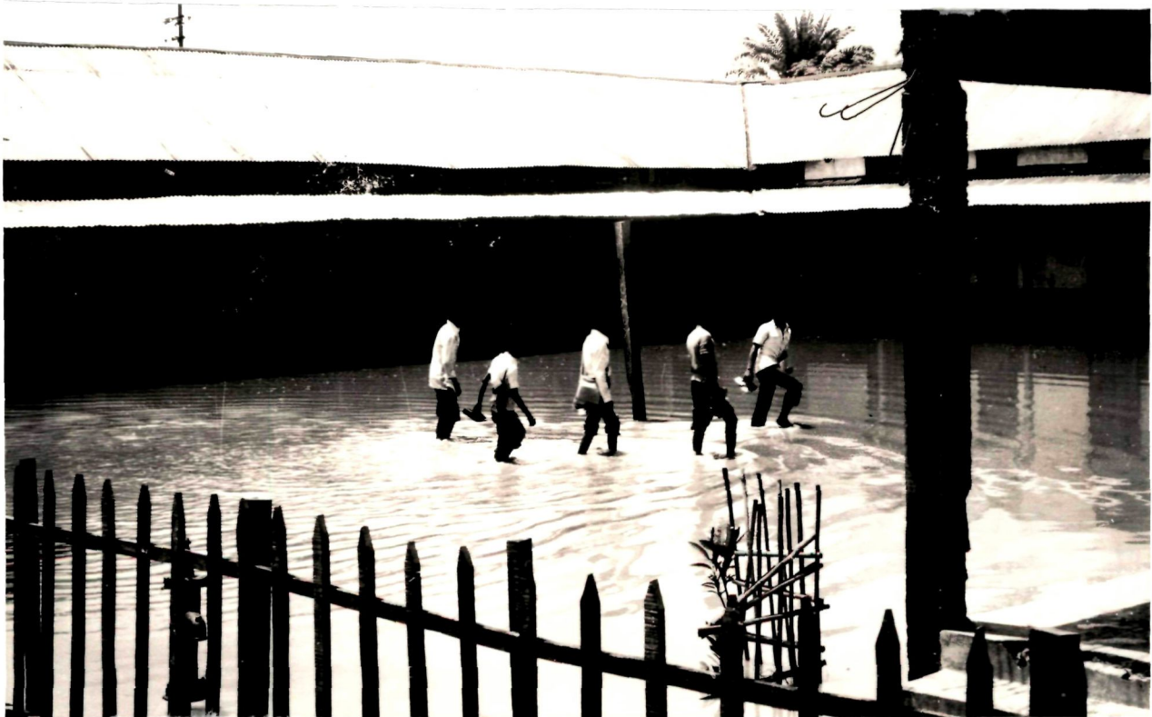
Plate 3: A tragic view of Bhaskar Vidyapith High School after heavy rainfall.
