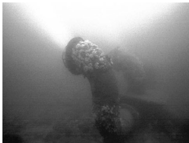
Fig. 8 Leaked effluents carrying pipe
