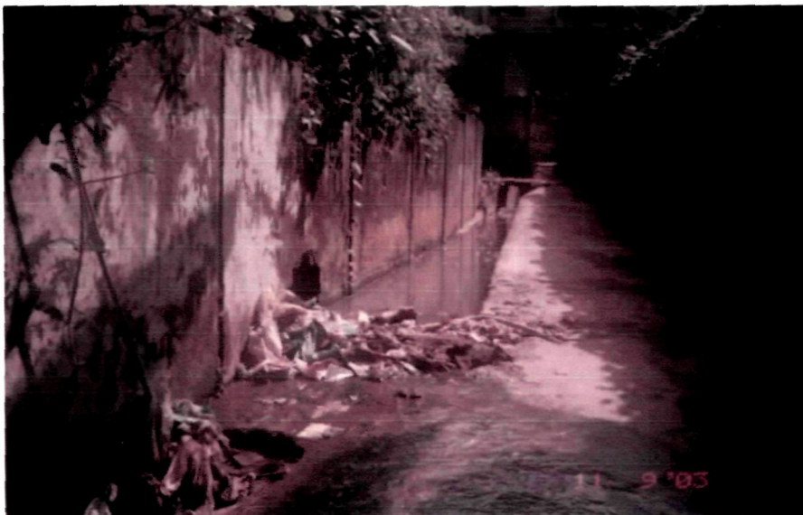
Plate 6.9 Street drains clogged with garbage.
